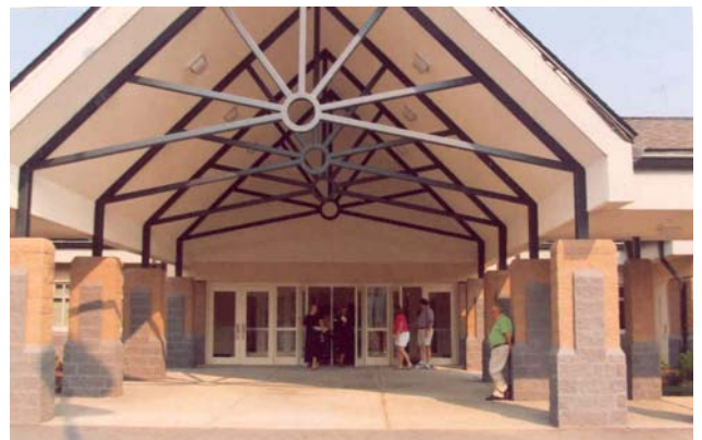
Main entrance to the new Robert L Patton High School.
